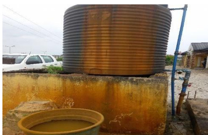
Fig.1: A typical impact of Fe in raw water on a surface in Bayelsa State
